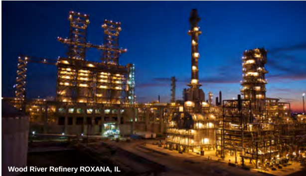
Wood River Refinery ROXANA, IL
