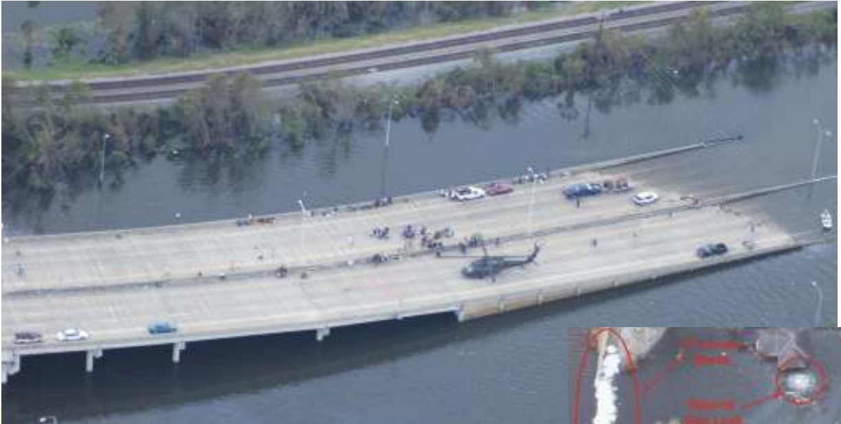
A helicopter conducts rescue operations on a partially submerged interstate.
