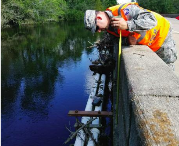
Lt. Col. George Stanley, commander of the South Carolina Wing's Sumter Composite Squadron, takes a high-water-mark measurement on the Sen. Roger W. Scott Memorial Bridge at the Little Pee Dee River in the wake of Hurricane Florence.
