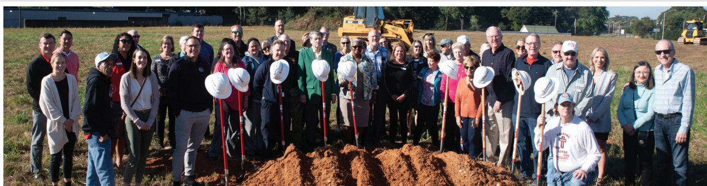
Good News at Noon recently broke ground on a new transitional housing shelter in Gainesville. The organization will use bunk beds it purchased with funds from a Jackson EMC Foundation grant for the new facility.
