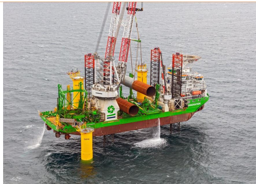
installation of first foundation for Dogger Bank A
