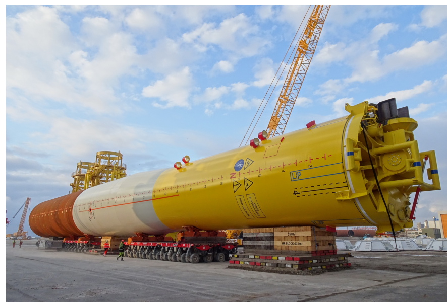
load-out of first monopile for Hollandse Kust Zuid
