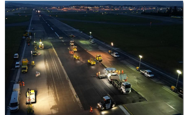
Refurbishment Runway 10/28 ~CHF 32 million
