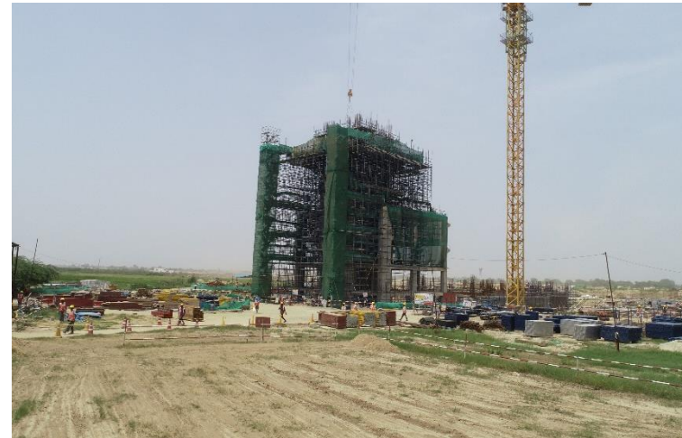
Air Traffic Control Tower
