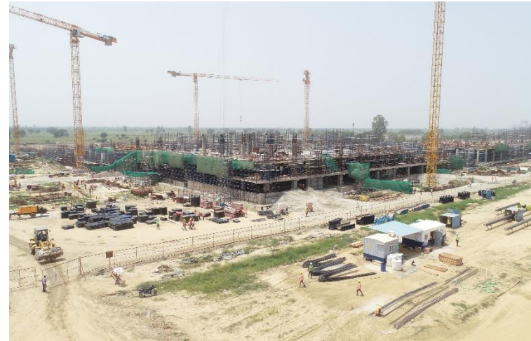
Passenger Terminal Building
