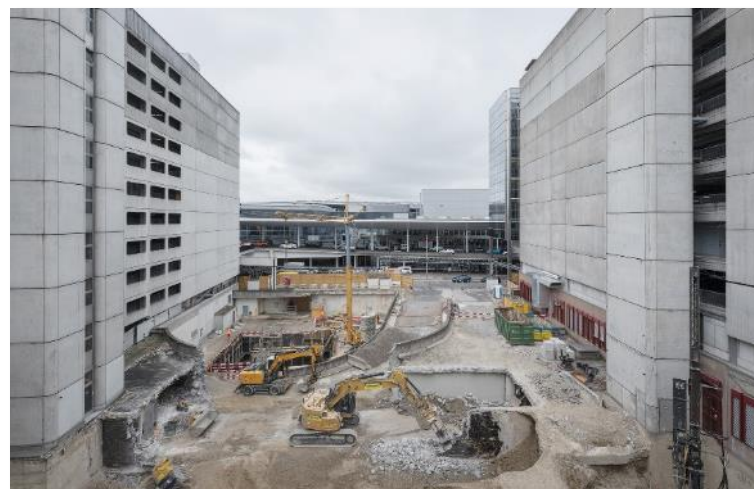
Development landside area ~CHF 14 million
