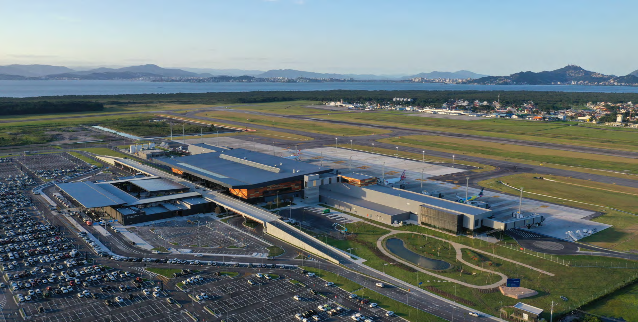
Florianópolis Airport – From old to new infrastructure in 16 months
