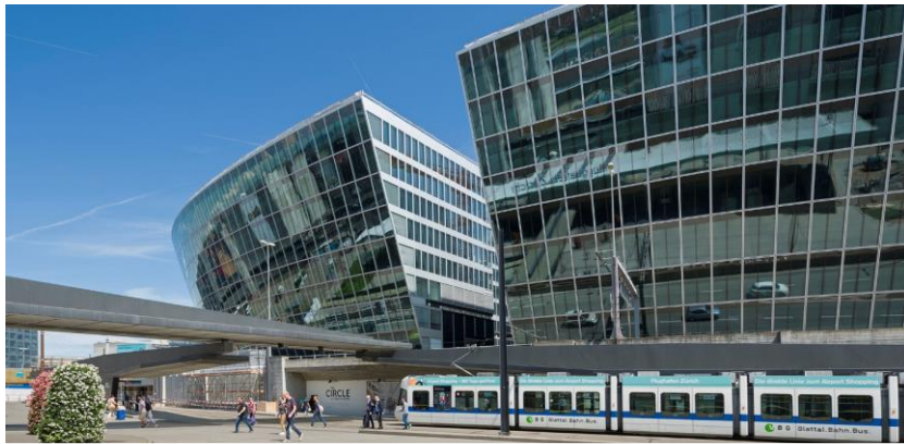
Core and shell is completed...
