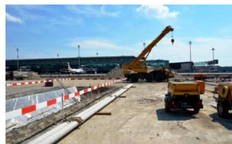
Civil engineering CHF ~30 million
