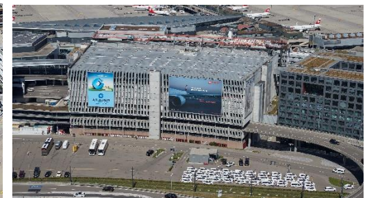
refurbishment P1 CHF ~10 million
