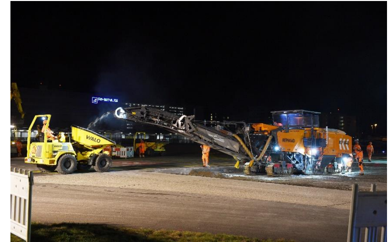
Refurbishment Runway 10/28 ~CHF 17 million
