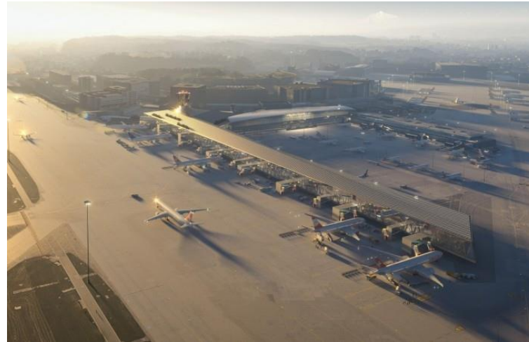
Pier with the gates
