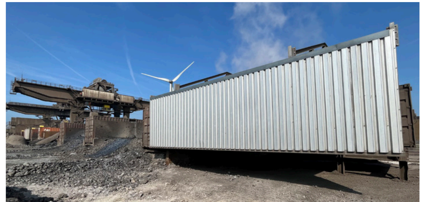
Less dust dispersion thanks to covered slag pits.
