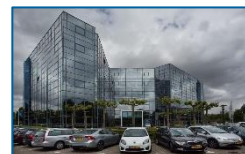
Park Office City: Rotterdam m2: 7,367
